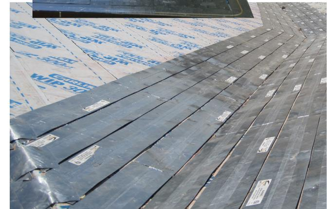
Tuff Cable can also be installed between strips of Heatizon Heatsink boards which have been screwed onto the sub-roof, then covered with Heatizon filler and bituthene.
